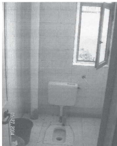
Toilet for persons with disabilities found in some courts
