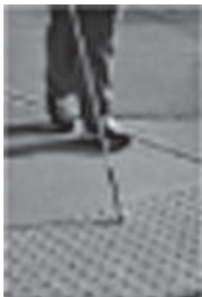
Model of rough tape that serves for the orientation of blind persons
